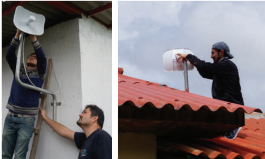
Figure. 5. Volunteers installing access networks. Own source.
