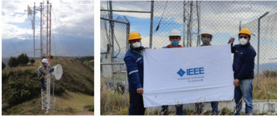
Figure. 4. Project team in the rehabilitation of the backbone network. Own source.
