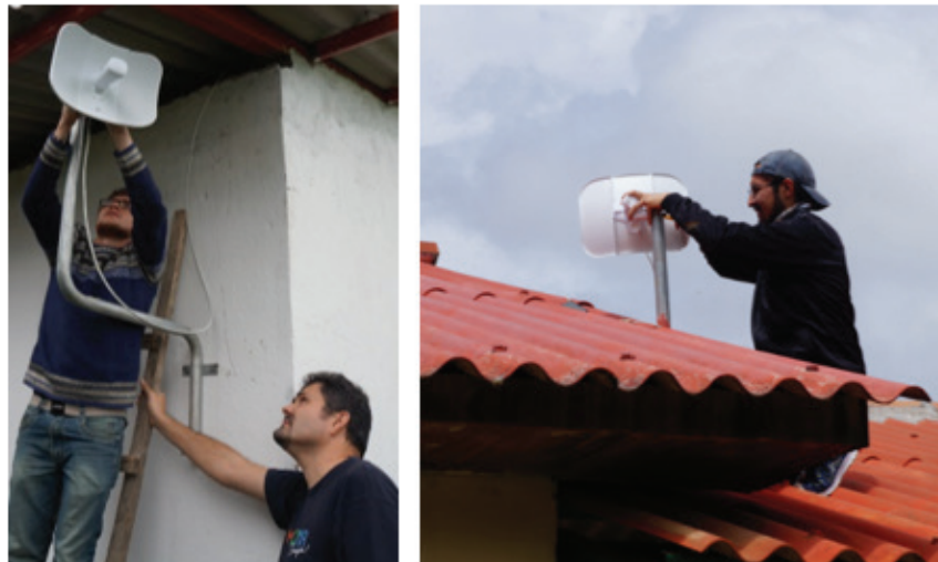
Figure. 5. Volunteers installing access networks. Own source.
