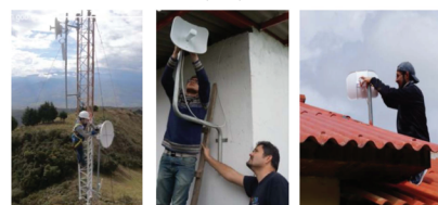
Fig. 5. Backbone and access network installation.
