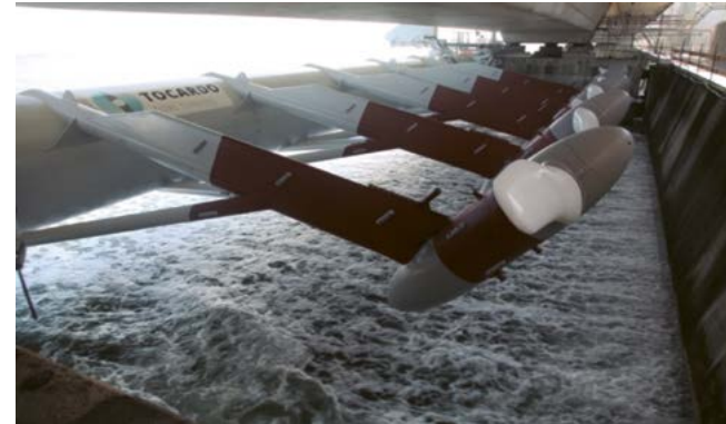
Fig. 1 Tocado Tidal Power 1.2 MW dam-integrated array
