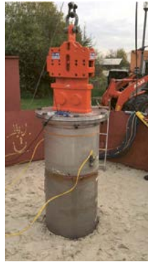
Fig. 2 Vibratory extraction with an Ape Model 3 vibrator of Cape Holland
