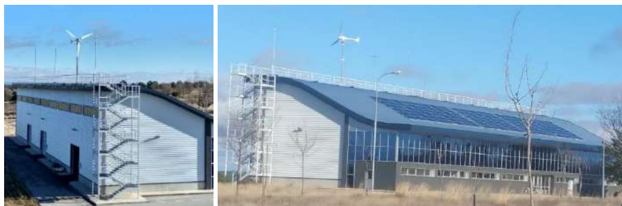
Figure 2. Enair EPRO70 Wind Turbine on the roof of LECA building.
