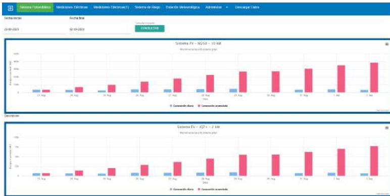
Fig. 5. View of the variables associated with the microinverters of the photovoltaic system
