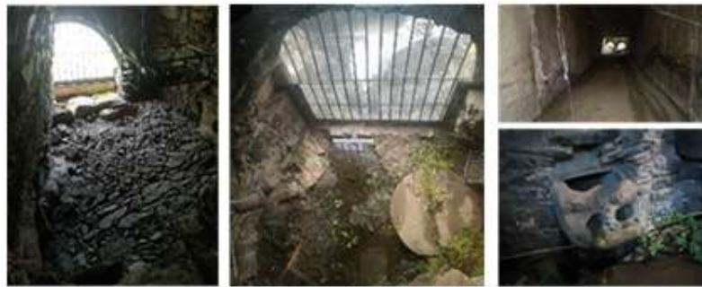
Fig. 2. Former mill infrastructures: two galleries and the water channel between them.
