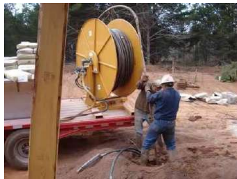
Fig. 3. Geothermal pipe-controlled descent. Comfortworks, Inc. Goldsby, Oklahoma, U.S.A.
