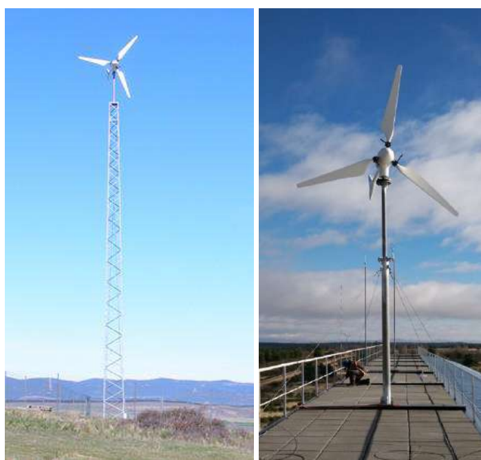
Figure 5. Enair EPRO70 Wind Turbine in an open field and peri-urban environment.
