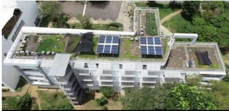
Fig. 1. GRIPV system of the Electrical Engineering building
