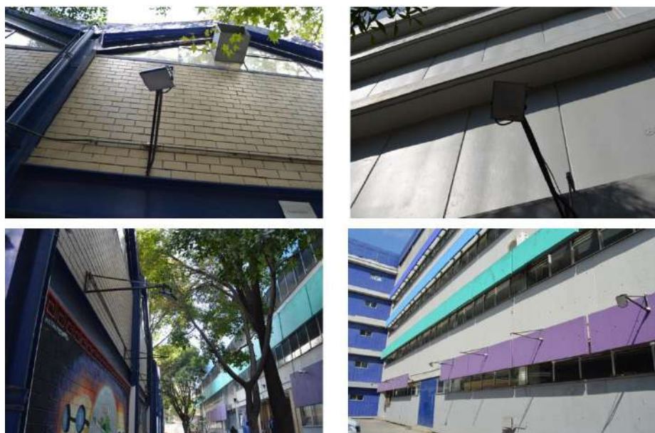
Fig. 5. Replacement of luminaires in EART.
